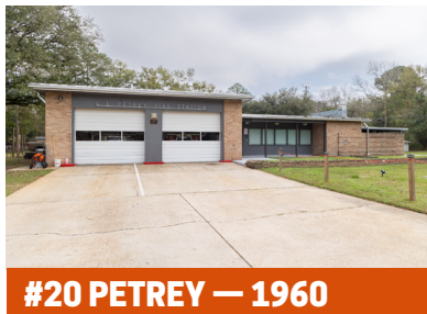
#20 PETREY — 1960 3471 Dauphin Island Pkwy Engine 20, Marine 20
