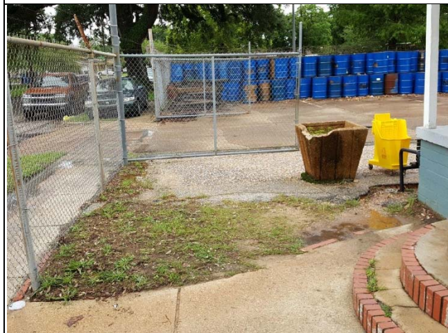
3. South Jefferson street entrance and concrete paved parking areas at the south side of the Eastern Maintenance building.
