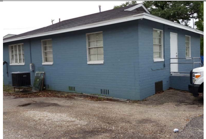
2. View of the Eastern Maintenance building.
