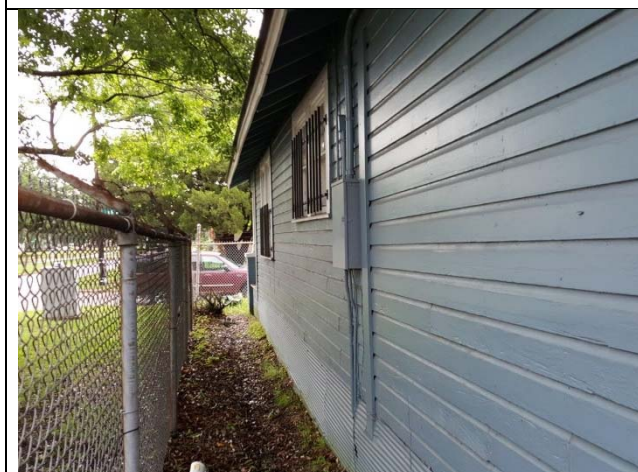
5. Exterior sidewall system at the Landscaping Services building consists of painted wood siding.
