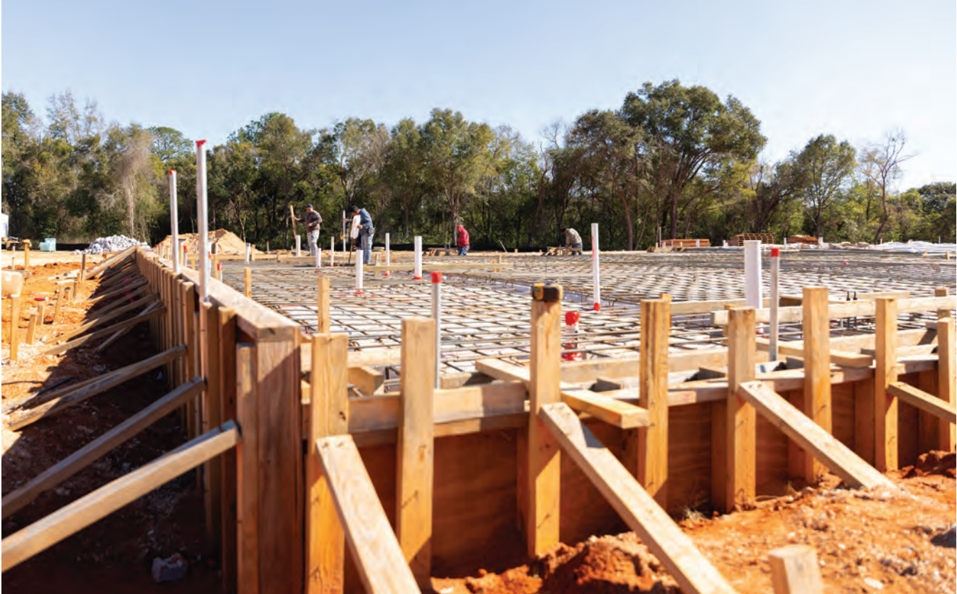
Progress photo of the foundation for the new McCosker Fire Station #19
